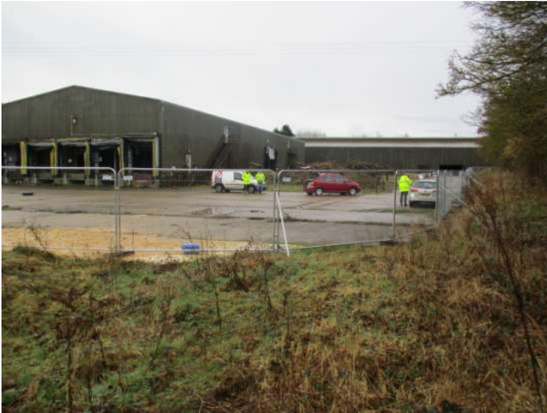
Plate 1. View of the site (looking west)
